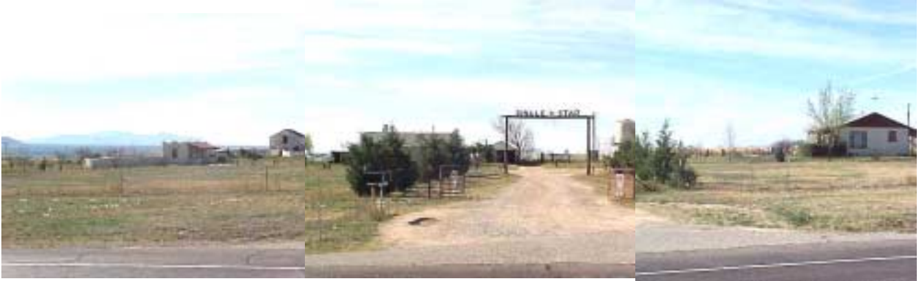
Typical Ranch style clustering of buildings: Preferred building massing is similar to historic ranch sites found throughout Cochise County—primarily one-story buildings clustered with view corridors between buildings and open expanses around buildings.
